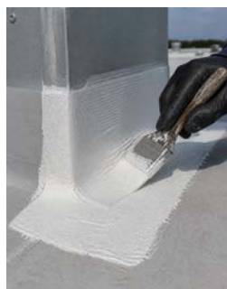
CURB FLASHING
