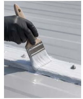
METAL ROOF SEAM + LAP
