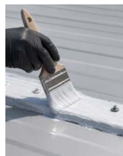
METAL ROOF SEAM + LAP
